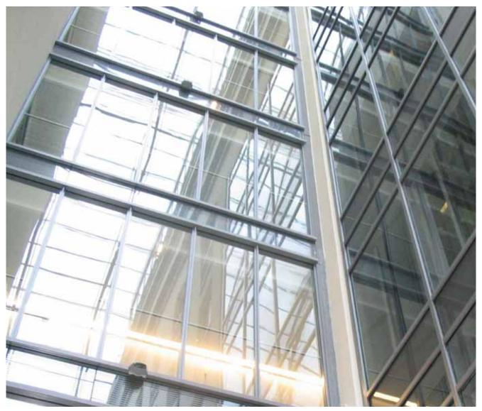
PYRAN® Platinum fire-rated glass-ceramic is tested and certified to stop the spread of smoke, hot gas and flames in fire-protection rated windows and transoms. During a fire, the glazing remains intact and transparent, allowing escaping occupants to clearly see the appropriate exit routes.
